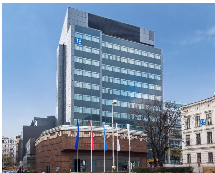
The Technical University Vienna has retrofitted its building at Getreidemarkt to a Passive House. The energy demand decreased from 804 to 56 kWh/(m 2 a). At the same time it produces 61 kWh/(m 2 a) renewable energy. Photo: Schöberl & Pöll
